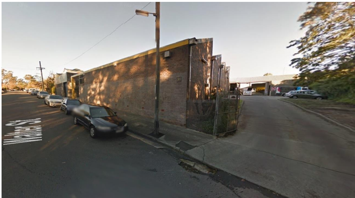
Figure 7 – Photo of the subject land from Walter Street (looking west)
